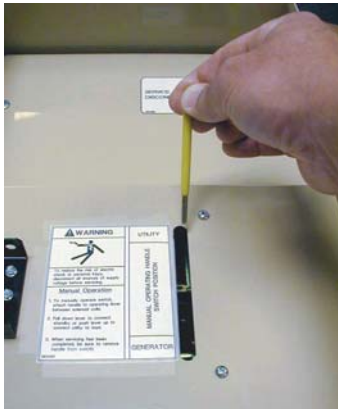
Figure 3.1 — Actuating Transfer Switch
